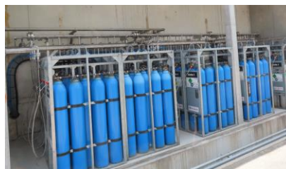
Figure 11 : New CH 4 -H 2 storage
