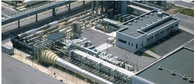
Fig 9. CIRA PLASMA TESTING complex aerial view
