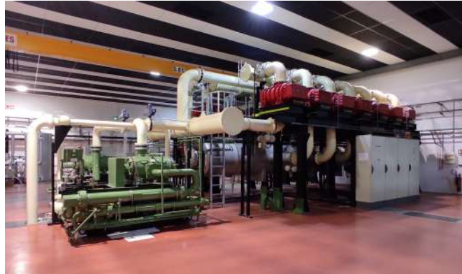
Fig 3. Wind tunnel MARHy pumping group
